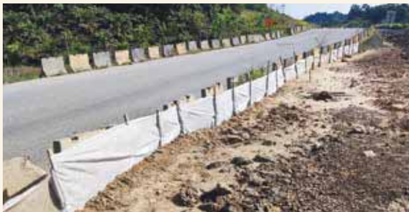
Silt fence on the Pan Borneo Highway
