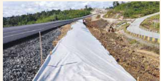
Silt fence on the Pan Borneo Highway
