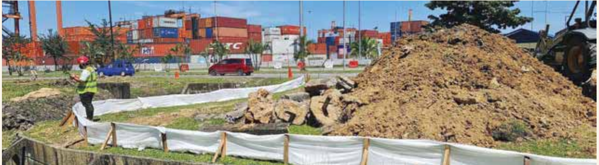
Silt fence at Container Port
